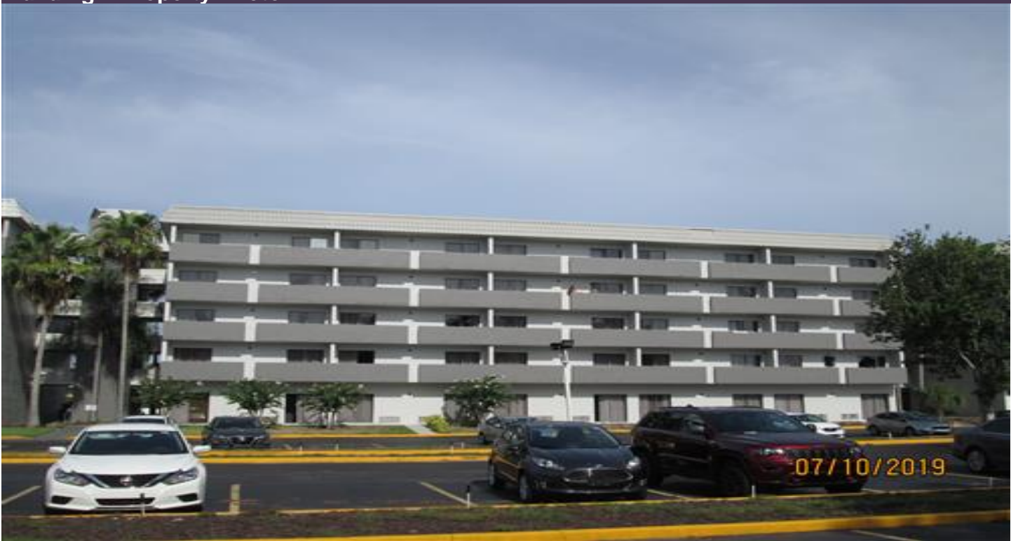
Building 2 Property Photo
