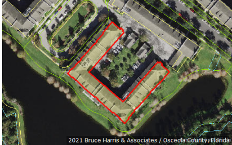
2021 Bruce Harris & Associates / Osceola County, Florida
