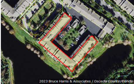
2023 Bruce Harris & Associates / Osceola County, Florida
